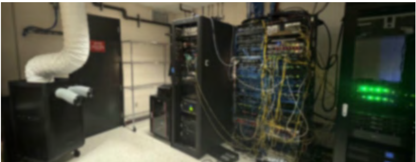
City server room with supplemental AC unit located to the left. Due to fire suppression requirements, hot air pulled from the room is pumped into the ceiling instead of being vented to the outside (Note : This image has been intentionally blurred for security reasons)
