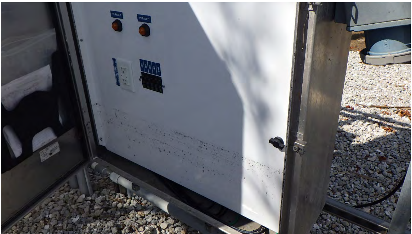
Wastewater lift station control panel with high water mark from Hurricane Ian
