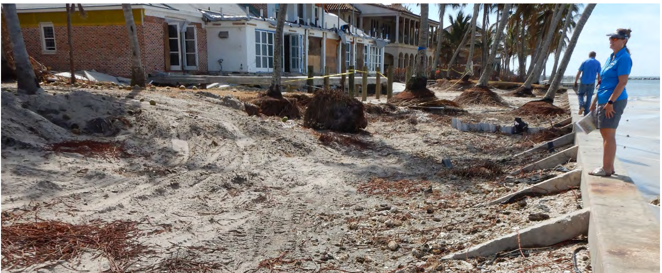
Seawalls overtopped and scoured during Hurricane Ian
