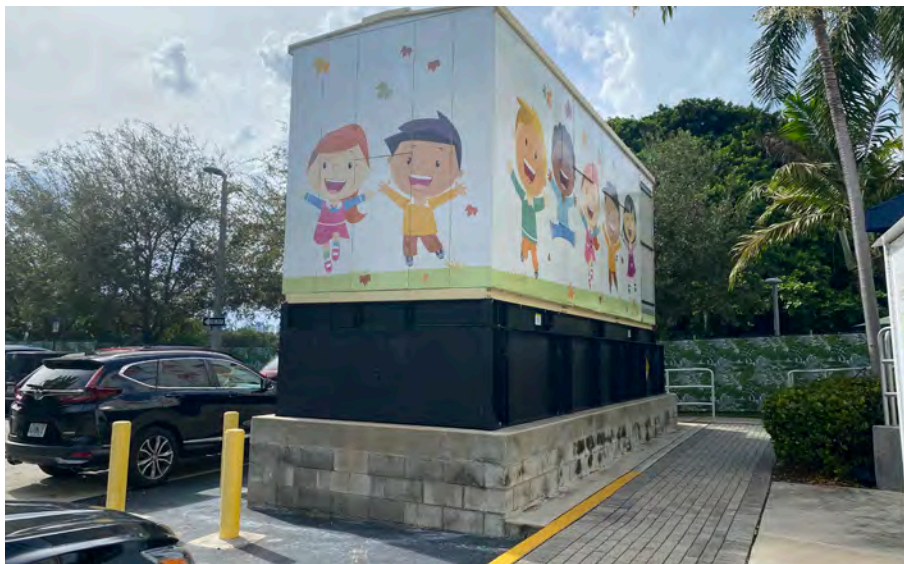
Elevated backup power generator for a community center in Miami Beach, FL
