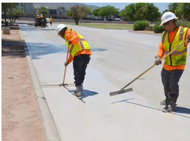
Workers applying cool pavement coating to roadway in Pheonix, AZ. Source: Scientific American
